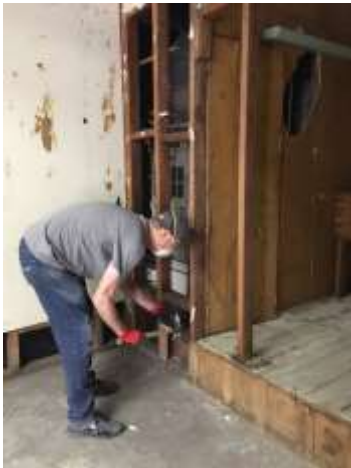
Rev. Dr. Patrick Horn helping by removing protruding nails and more.
